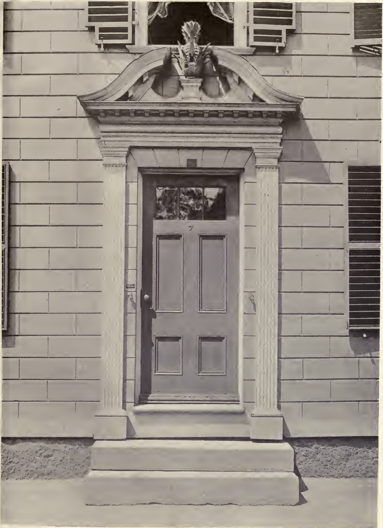
PINEAPPLE DOOR BROWN STREET, SALEM, MASS. SAMUEL McINTIRE, ARCHITECT
